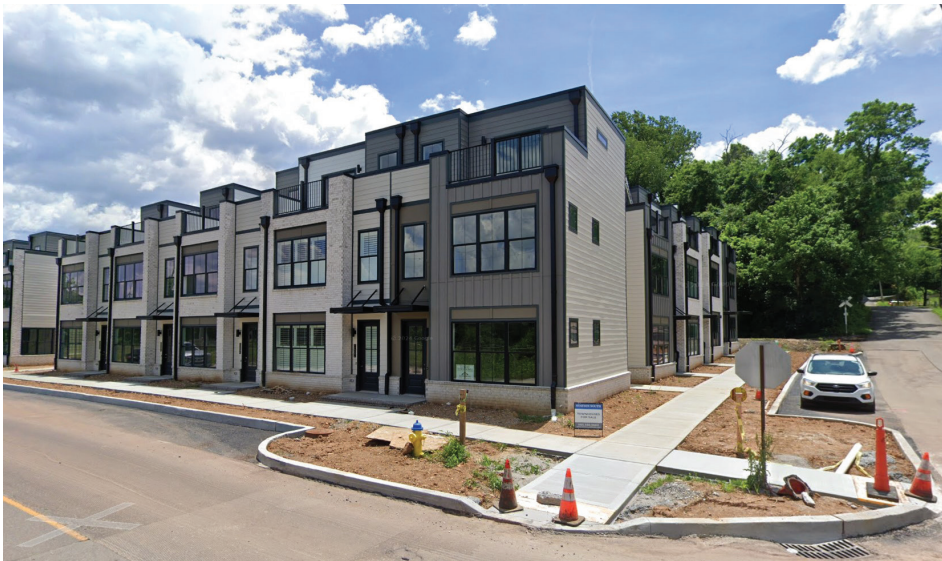
1400 Island Home Ave - Tailwater South
